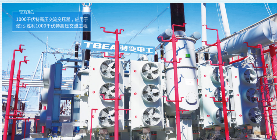
Figure: A 1,000kV UHV AC transformer, is applied in the Zhangbei-Shengli 1,000kV UHV AC project
